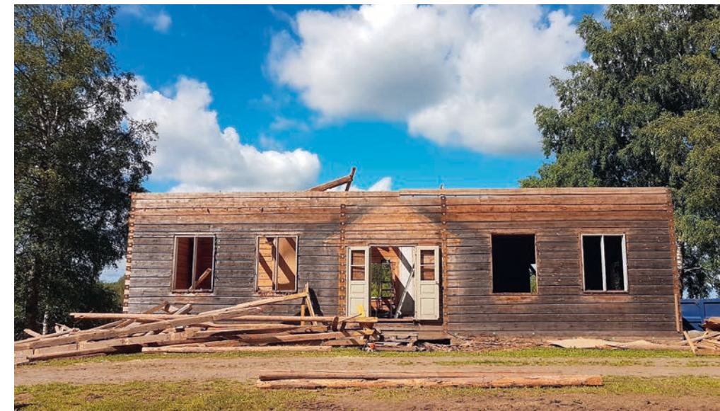
Hirsitalo, jonka kattorakenteet on purettu. | Log house with dismantled roof.
