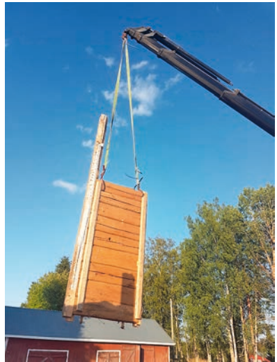
Hirsielementin nosto | Lifting a log element
