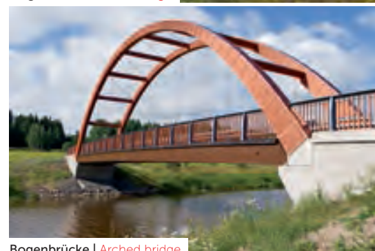
Bogenbrücke | Arched bridge
