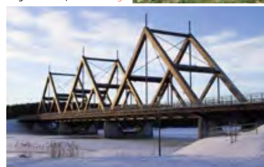
Brücke in Verbundbauweise | Crossed-stressed bridge
