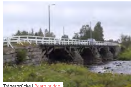
Trägerbrücke | Beam bridge
