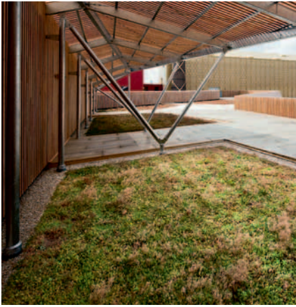
Casarès-Doisneau inter-municipal school complex Sijainti Location: 3, Rue Cristino Garcia, Saint-Denis 93
