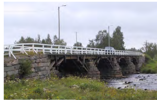
Tukiansassilta | Beam bridge
